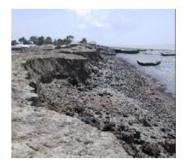
Besides the erosion of the riverbanks, the foreshore and the embankment systems are posing a continuous problem in the coastal areas. This exposes interior lands to the threats of cyclone surges and salt-water intrusion.
